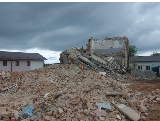
Image 2 Demolition of the hospital's main building, a Habsburg era military
