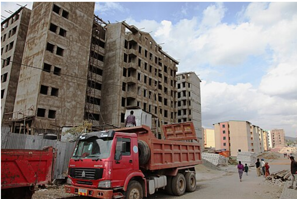
New homes and residences are being built around Ethiopia's capital, Addis Ababa. By DFID - UK Department for International Development , courtesy of Wikimedia Commons .
