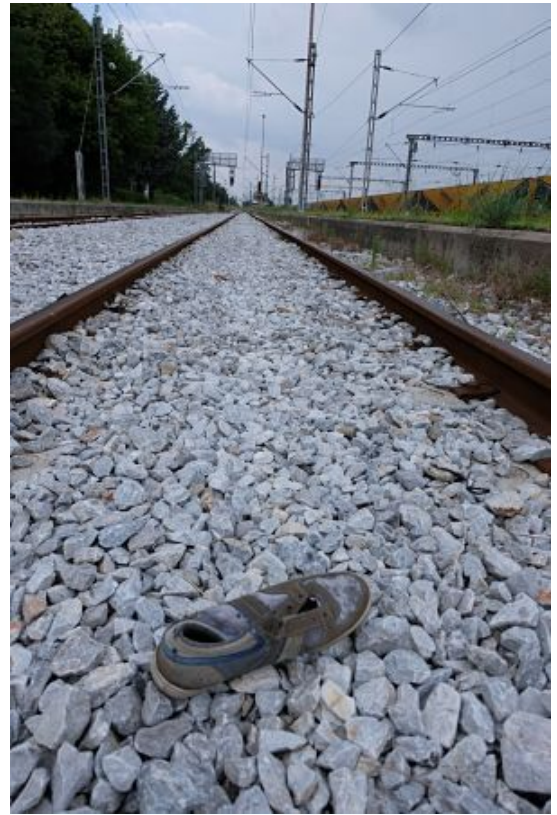
Idomeni railway station on the border between Greece and Macedonia, July 2017
